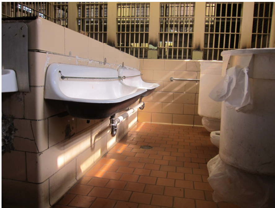
(Kilby Dormitory A bathroom, showing garbage can on top of accessible toilet)
