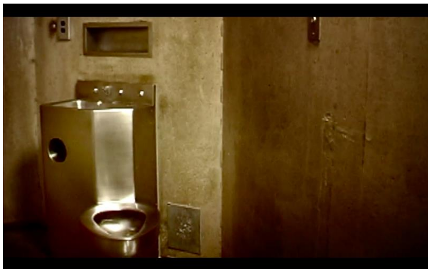
Figure 2 Sink and Toilet
